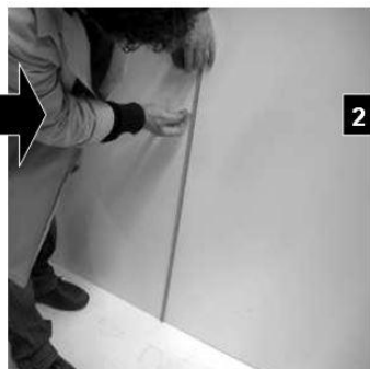
1 Determine the finished height
