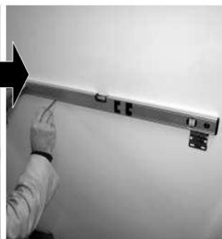
4 Place the second wall plate aligning it with the first one
