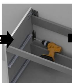
2 Fixing the brackets on the unit
