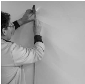
1. DETERMINE THE FINISHED HEIGHT
