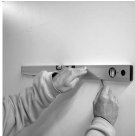
4. FIX THE SECOND SCREW ALIGNING IT WITH THE FIRST ONE
