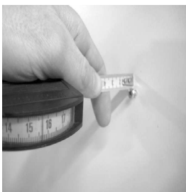
3. THE SCREW MUST PROTRUDE MAXIMUM 8 MM FROM THE WALL
