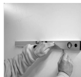
4 Place the second screw aligning it with the first one
