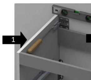
1 Adjust the level of the unit
