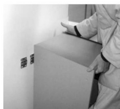
1 Hang the unit on the wall plates
