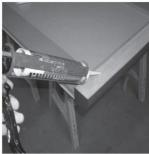
We recommended a silicone spot on each rear  $\underline{bottom\ corner\ of\ the}$   $\underline{mirror}$
