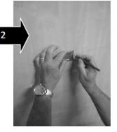
2. Position the wall plate, mark and drill
