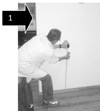
1 Determine the finished height
