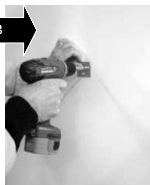
3 Fix the first wall plate
