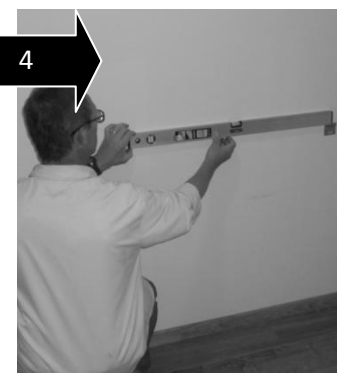
4 Place the second wall plate aligning it with the first one
