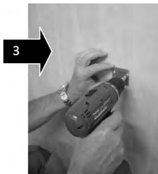
3. Fix the first wall plate
