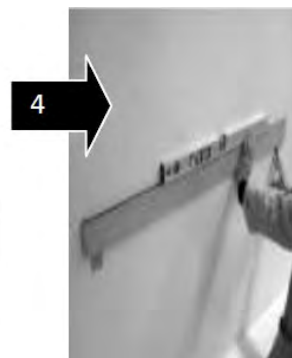
4. Place the second wall plate aligning it with the first one
