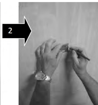
2. Position the plate, mark and drill
