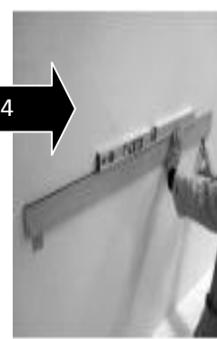
4 Place the second wall plate aligning it with the first one
