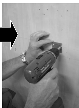
3 Fix the first wall plate
