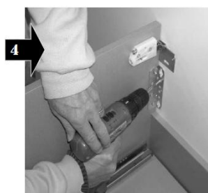
4 Fix the extra brackets to the wall (screw not provided)
